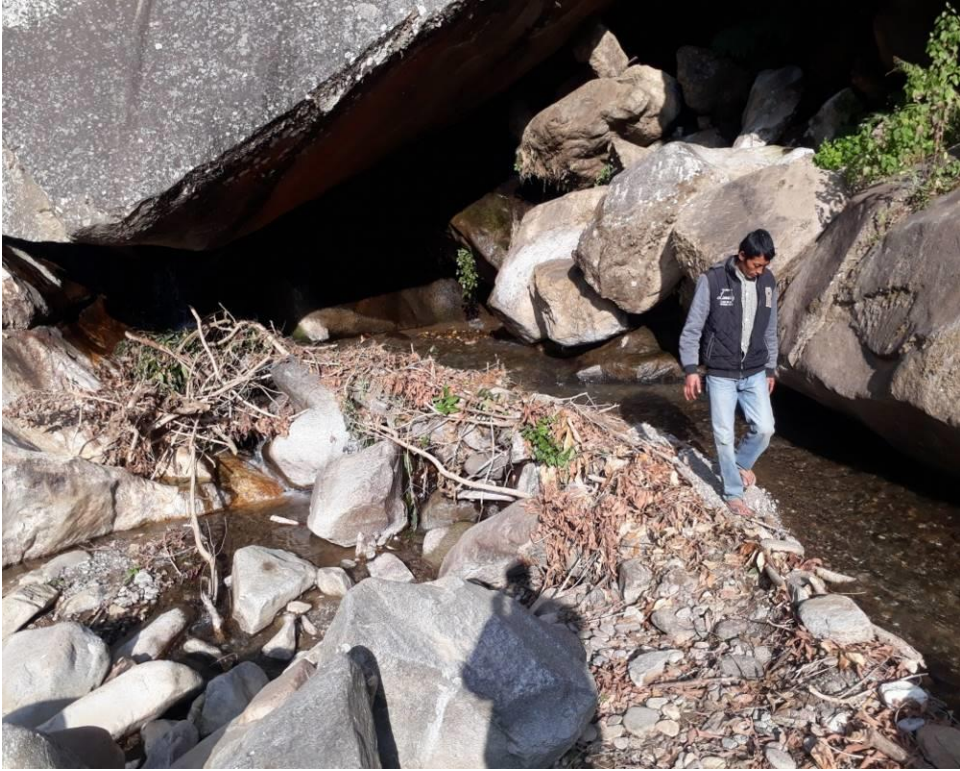
Picture 1: Temporary weir
